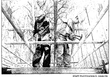
Carpentry students Paul Smith and Brian Wells remove nails to correct the roof truss centers on the BOCES building they are renovating behind the Forman Center. The building was damaged by an electrical fire last spring.
